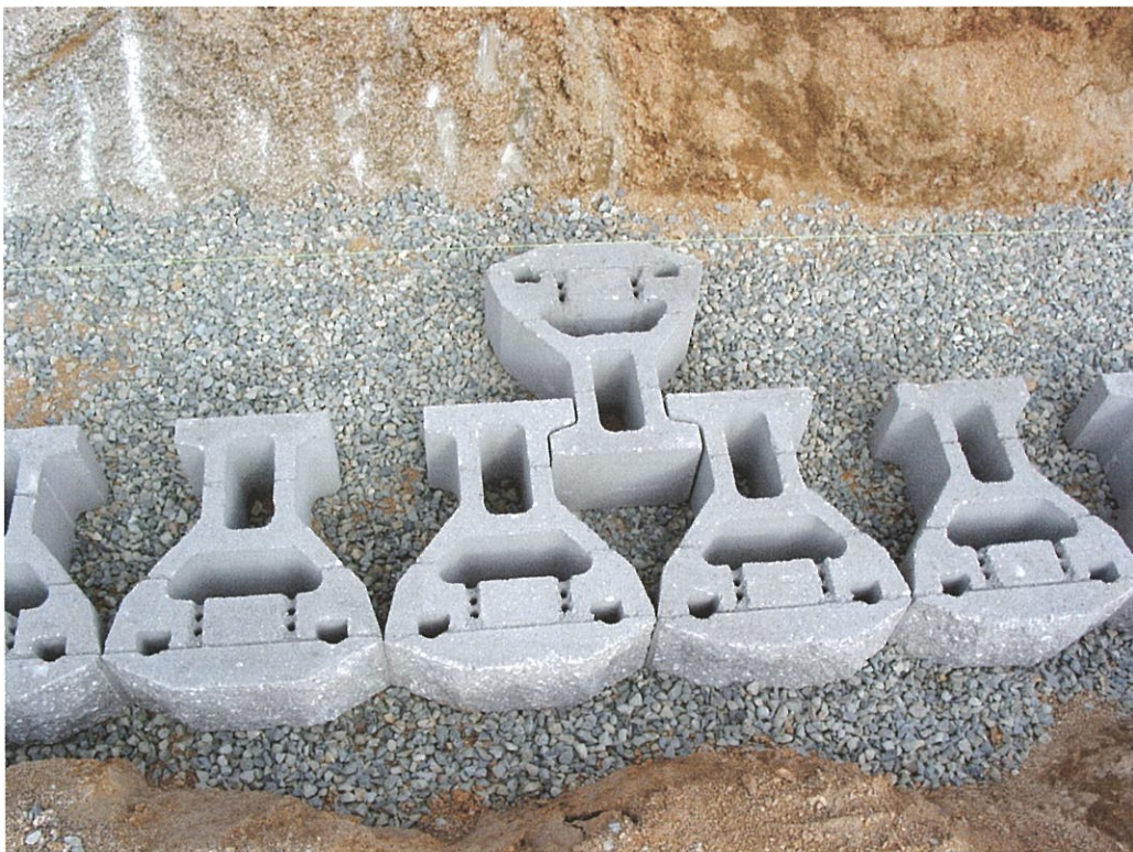
Initial Course of GeoWall Max on Leveling Pad
