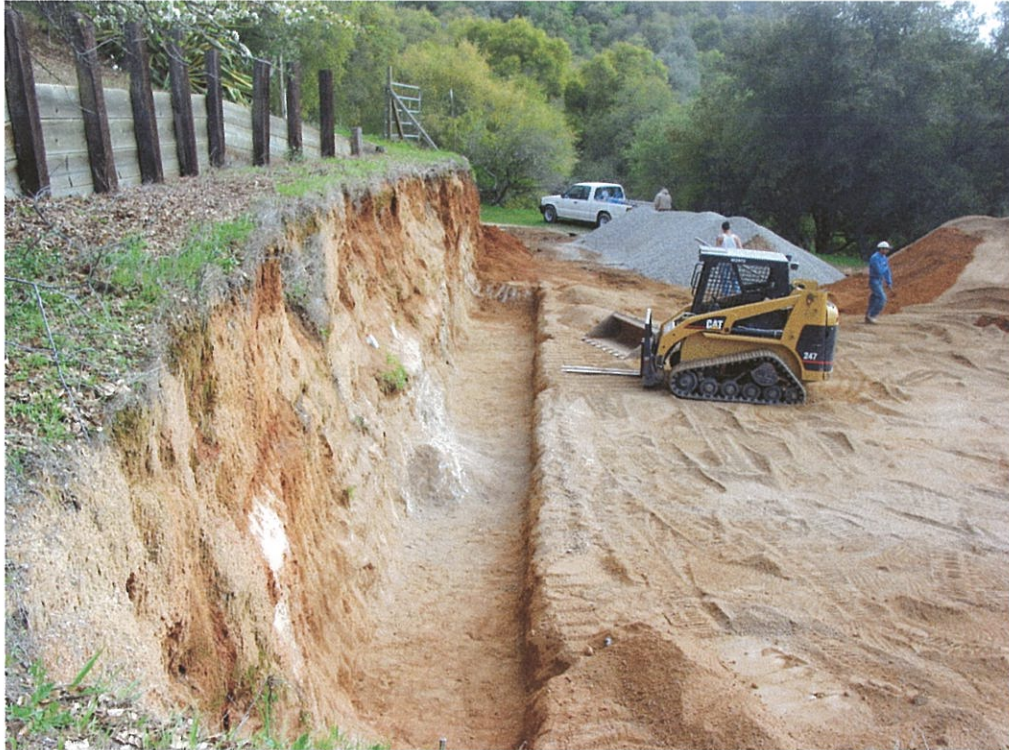
Subgrade Prepared for Leveling Pad
