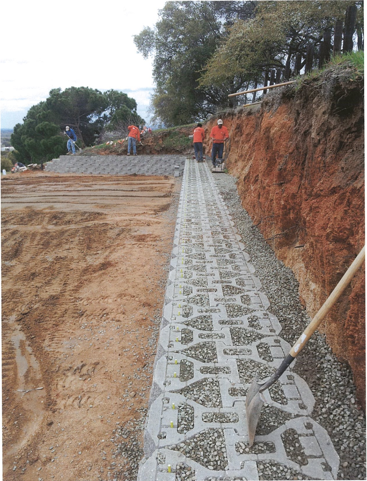
Two Courses Installed. Note Rear Pin Position for Installation.
