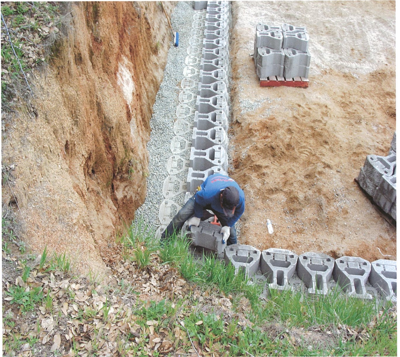
Drain Rock Installed as Blocks are Installed
