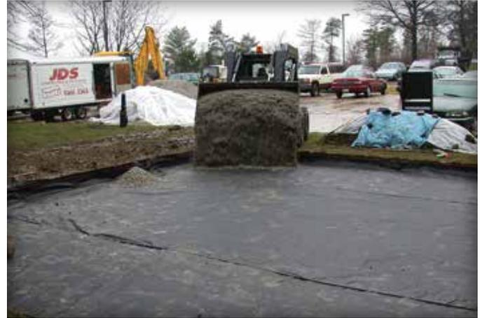
Figure 3. Application of the geotextile under aggregate base.
