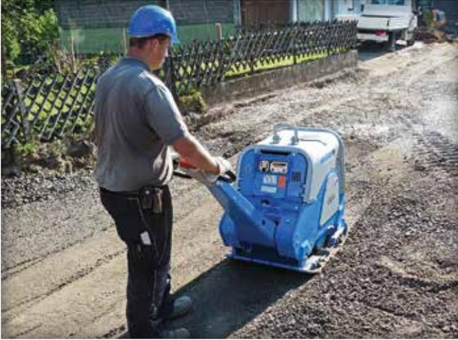
Figure 4. Base compaction with a reversible plate compactor.
