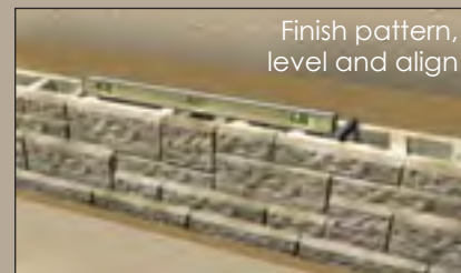
Compact on block and behind
