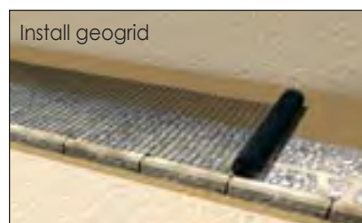
Install first course of pattern on top of geogrid
