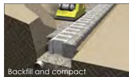
Install anchoring units
