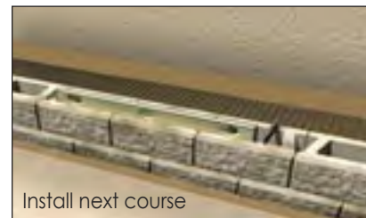
Install AB Reinforcement Grid
