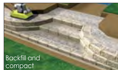
Install wall out from stairs
