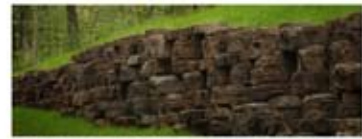
Grade slope to rise above top blocks, giving the look of natural outcropping in the bank. (Design must account for surcharge loading)
