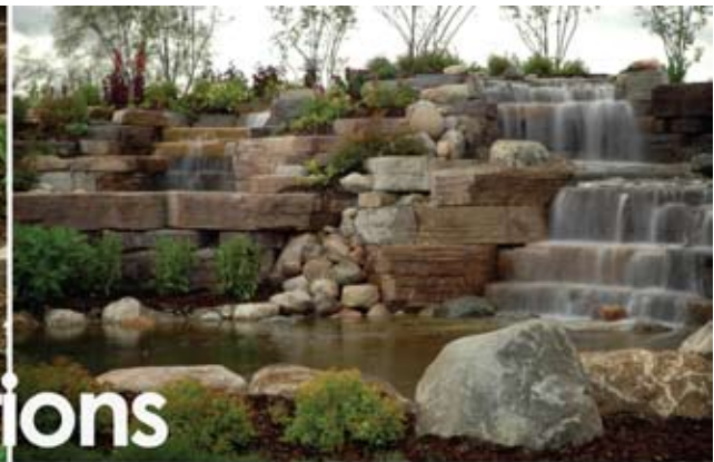
Grade slope to rise above top blocks, giving the look of natural outcropping in the bank. (Design must account for surcharge loading)
