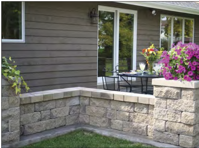
Built on existing foundation
