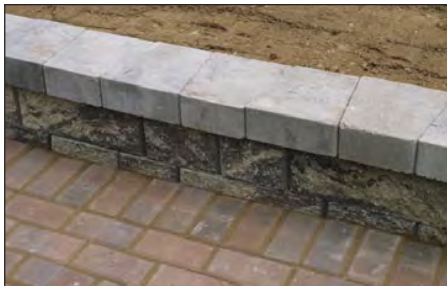
Compact soils with a hand tamper behind block
