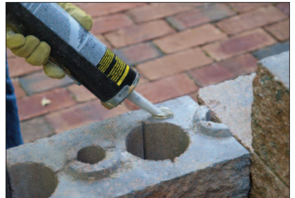
Use Adhesive to Secure
