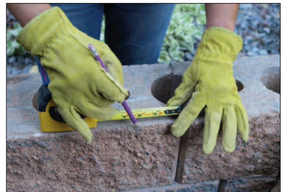
Mark and Cut Corner Block
