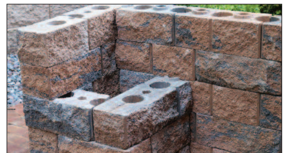
Mark and Cut Corner Block
