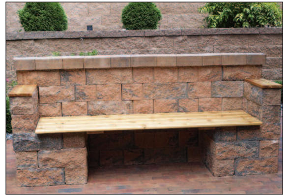
Install Seating Materials
