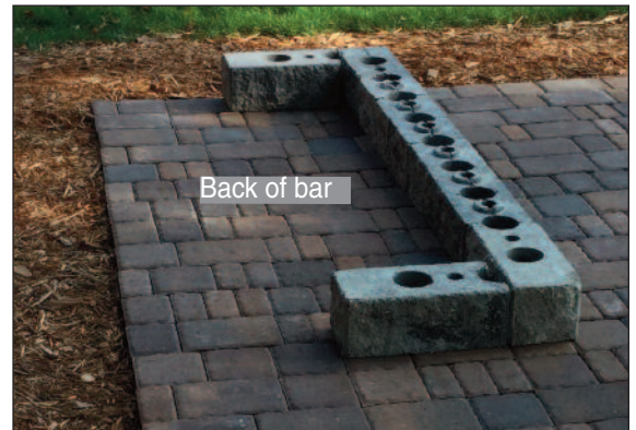
Build the First Course
