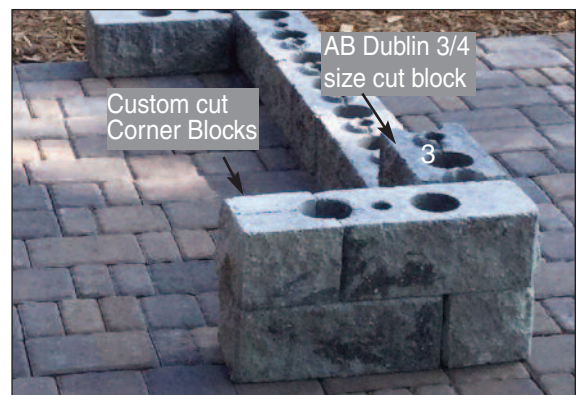
Start Back Wall
