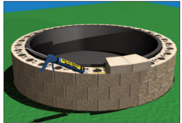
Install Liner and Caps
