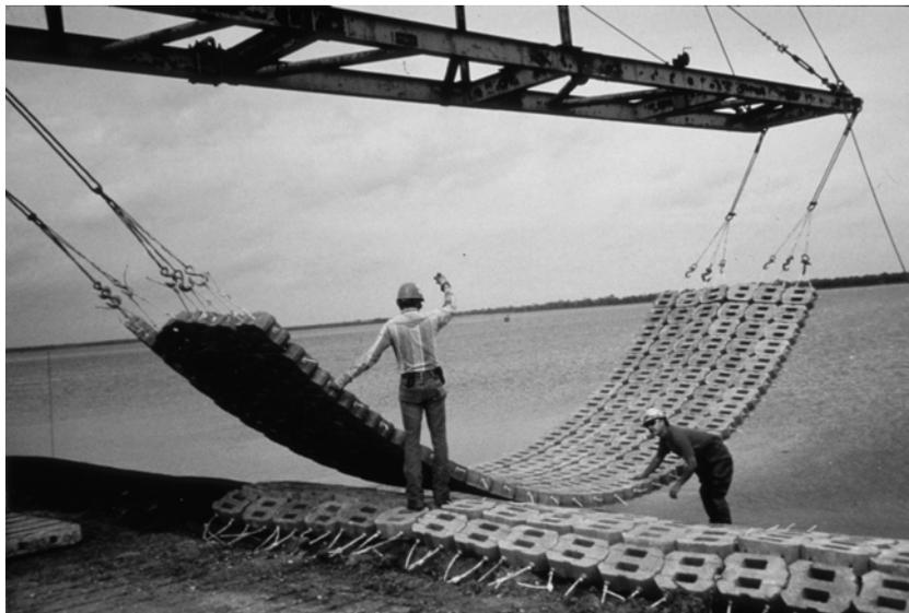
Figure 7.3: Close-up of spreader bar and ACB mat.
